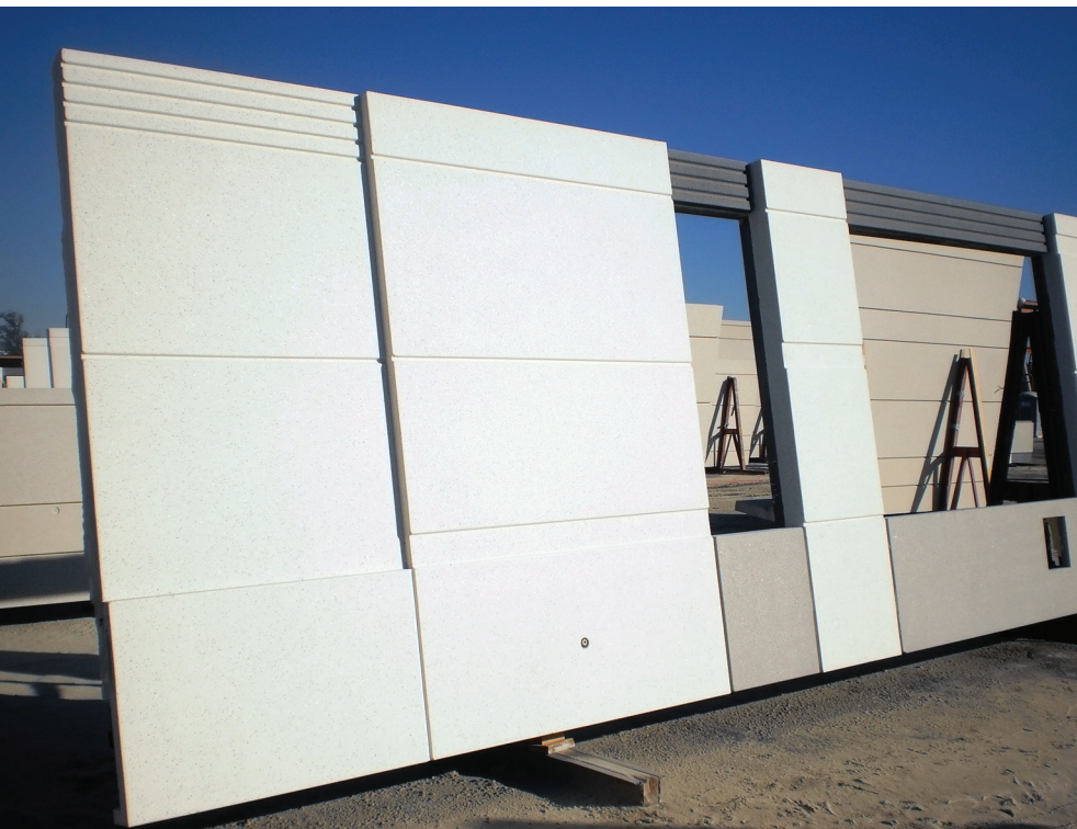
C-CAPP Panel with Architectural Finish ©Clark Pacific 2013
