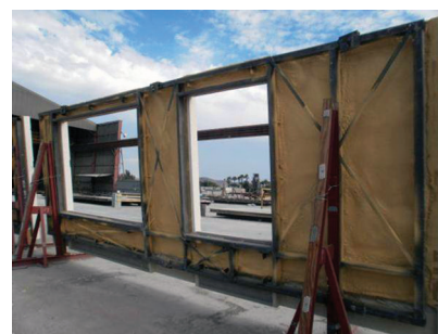
Interior Panel View with Spray Foam Insulation ©Clark Pacific 2013
