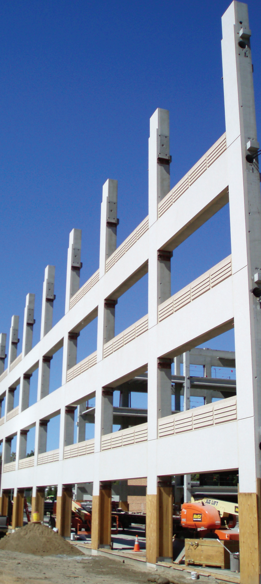
Detail of the Caltrans District 3 precast hybrid moment frame. Photo by Clark Pacific
