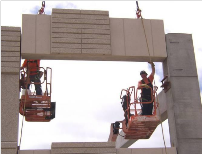
Precast Hybrid Moment Frame Beams
