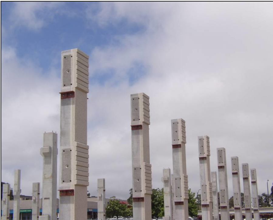
Precast Hybrid Moment Frame Columns
