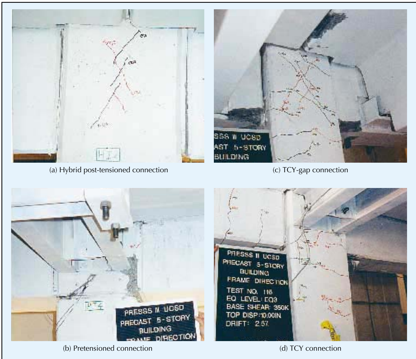
Fig. 16. Condition of frame connections after design level of response.
