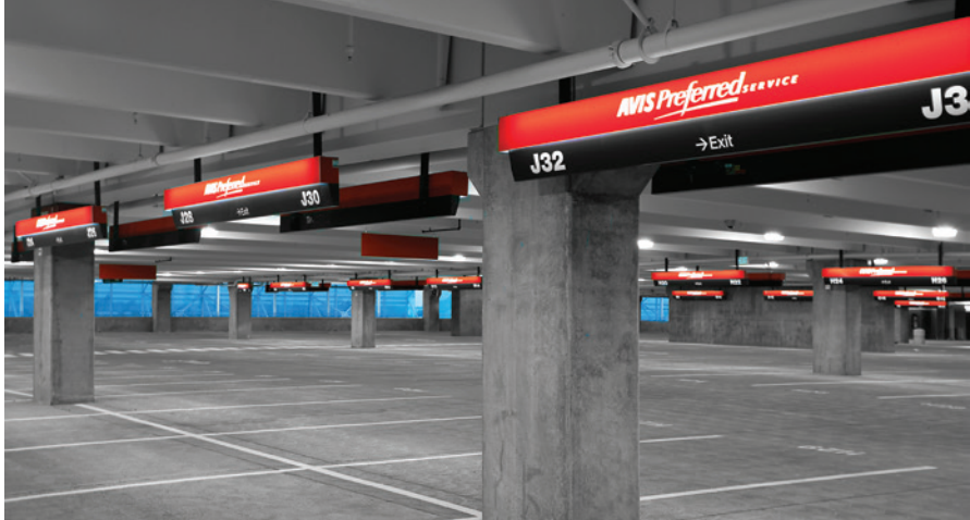
Half as many interior columns with long-span double tee solution vs. conventional cast-in-place construction.
